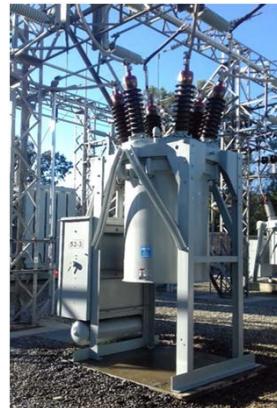
Typical Oil Circuit Breaker (Aged Unit)
