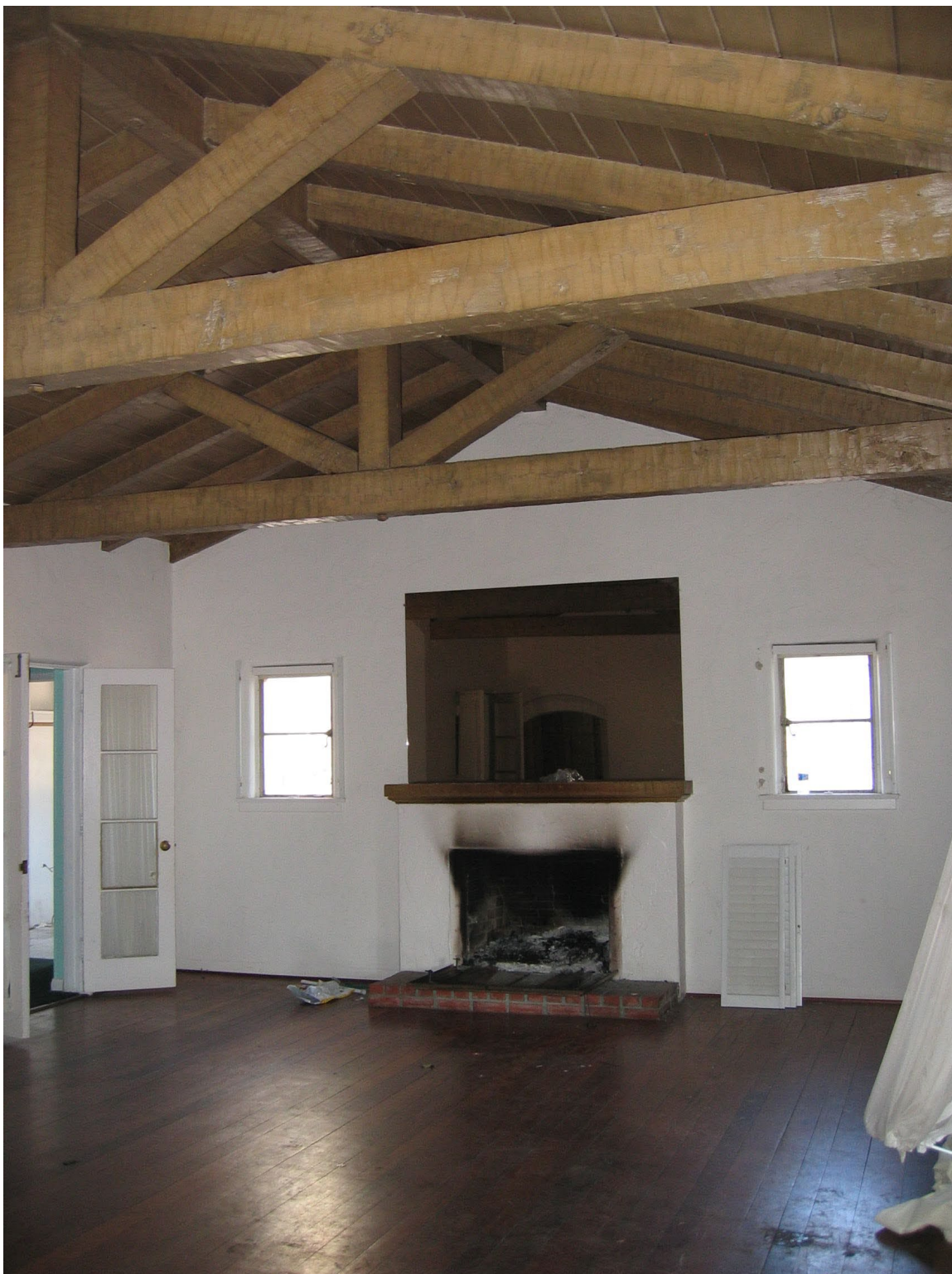
Figure 8 - Living Room Before Rehabilitation
