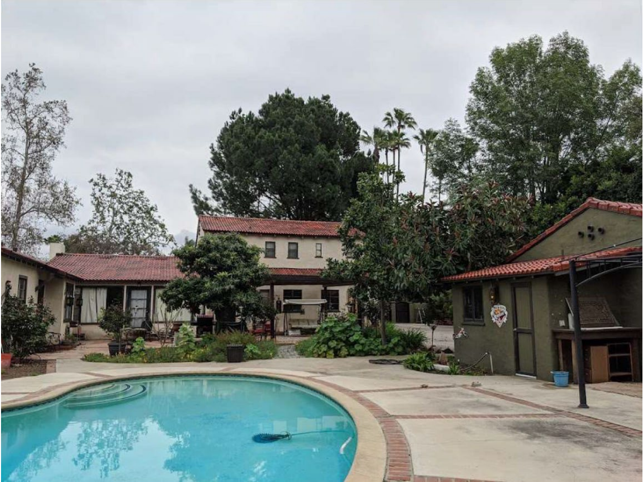
Figure 7 - Rear of the Residence - View Looking East
