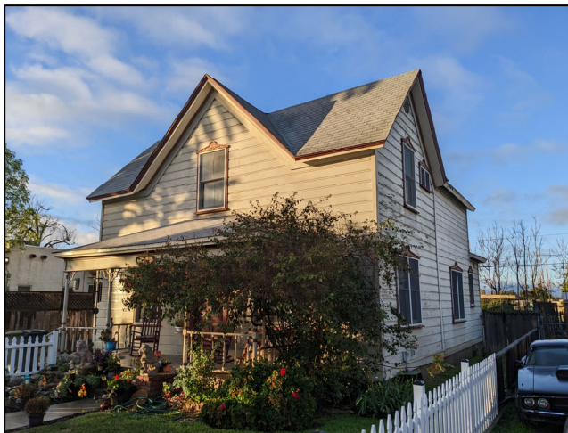
Northeast (Front) and Northwest (Side) Elevations
