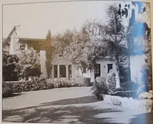
Rear elevation, Edward Doyle residence, sharing adjoining park-like backyard space with the Jekel-designed Arthur N. Sweet residence next door. A stone-clad lily pond stands prominently in the foreground, confirming Jekel's preference for water features in the landscapes of his houses.
