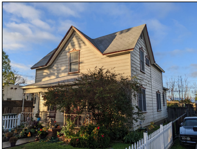
Northeast (Front) and Northwest (Side) Elevations
