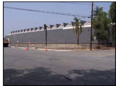
Plant 2 East Elevation, Looking Southwest; 2012
