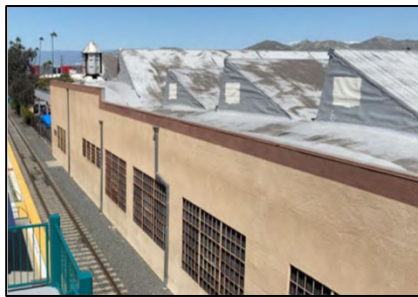
Plant 1 West Elevation, Looking Northeast; 2021
