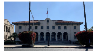
Maintaining 4 historic sites (7 sites total)
