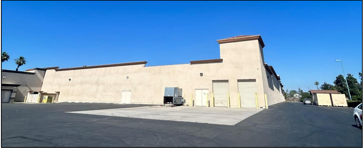
View of the existing site looking northeast from the parking lot.
