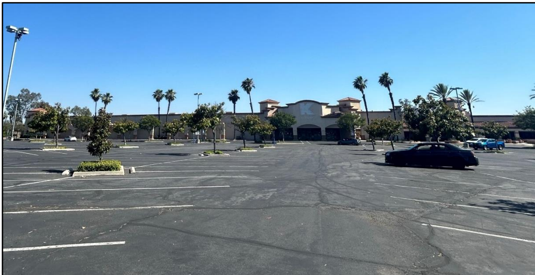
View of the existing site looking south from the parking lot.
