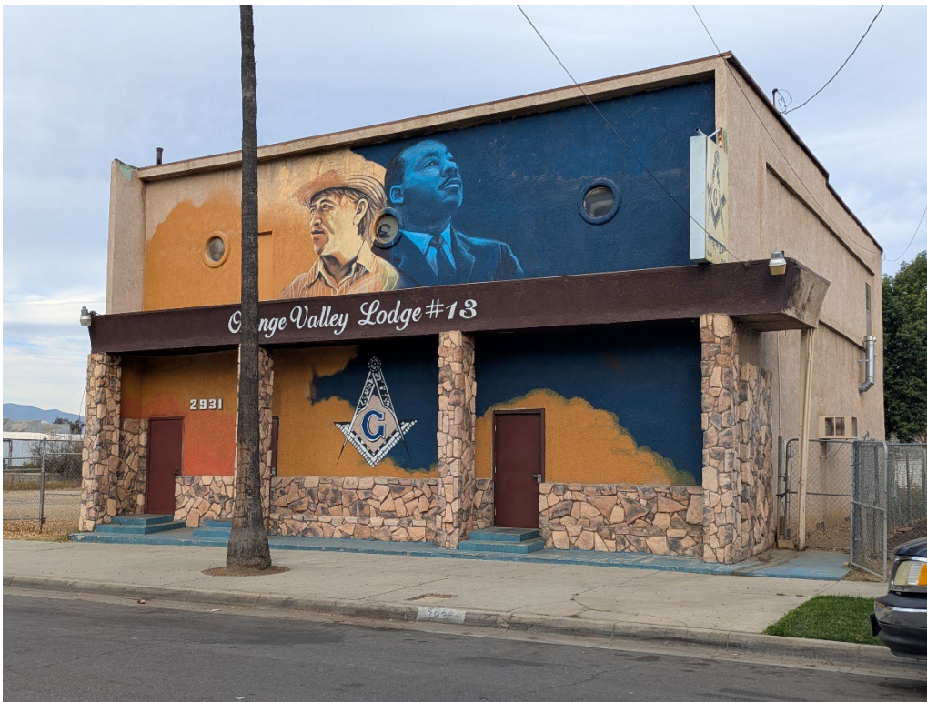
Figure 2 – Façade (South Elevation) and east elevation, view looking northwest
