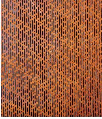
PERFORATED STEEL HUES OF RUSTED RED & BROWN OCCURS AT STAIR TOWERS - ALL LEVELS
