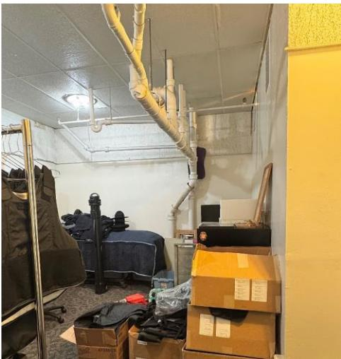
**Water and sewer lines** running along/above electrical components are found throughout the building.
