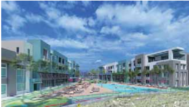
VIEW TO POOL AREA
