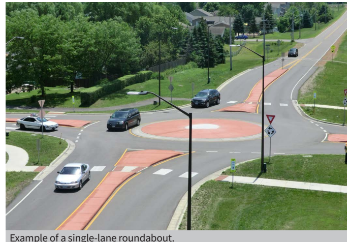
Example of a single-lane roundabout.
