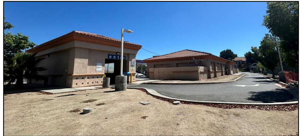
VIEW FACING NORTHEAST FROM SOUTH PROPERTY LINE
