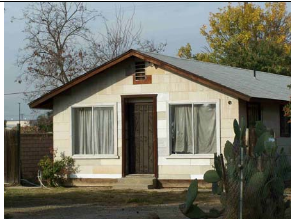
Figure 28: View looking northwest at the post-war era asbestos asphalt shingle cladding and replaced windows of 7771 Janet Avenue
