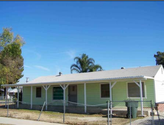
Figure 25: View looking northeast at 8022 Cypress Avenue
