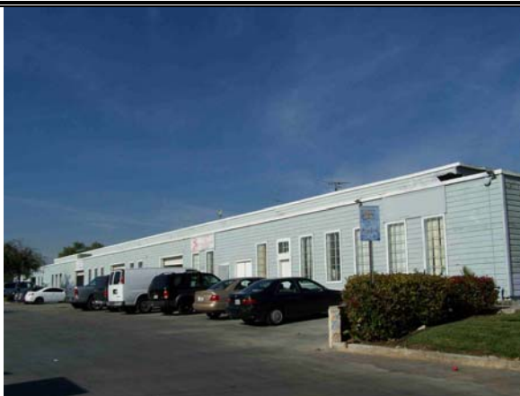
Figure 41: View looking northwest at the laundry facility
