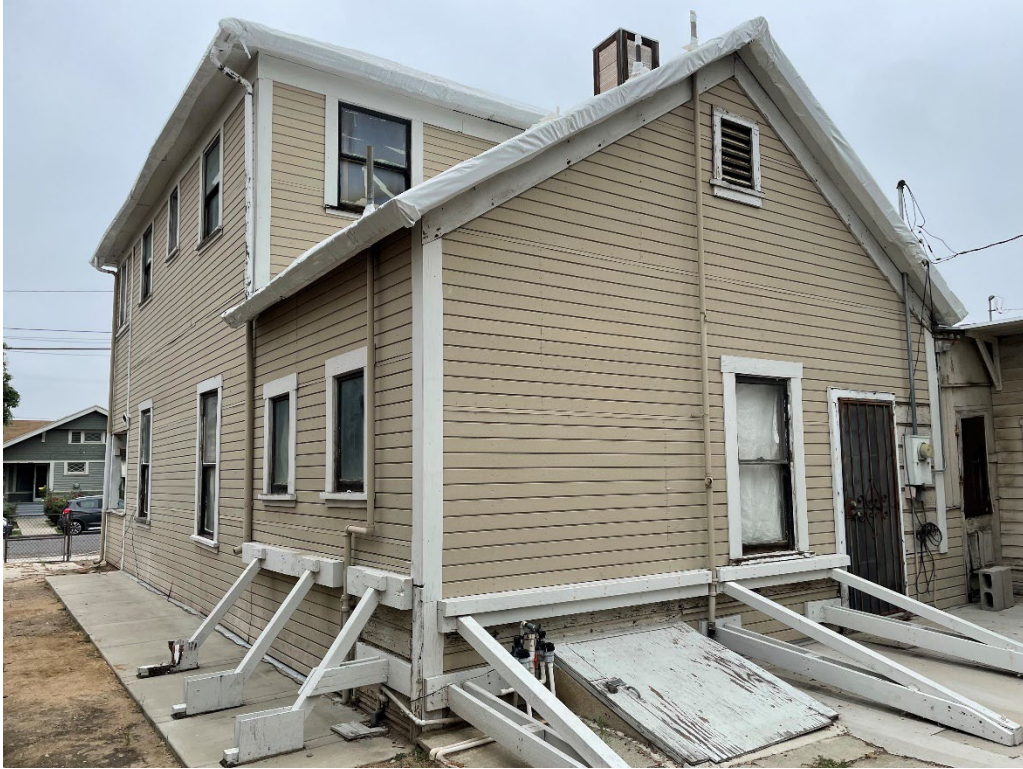
Figure 5 - Harada Hose east (rear) elevation, view looking northwest
