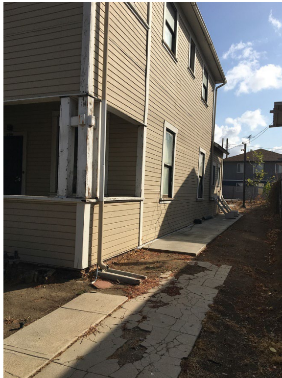
Figure 4 - Harada Hose south elevation, view looking east
