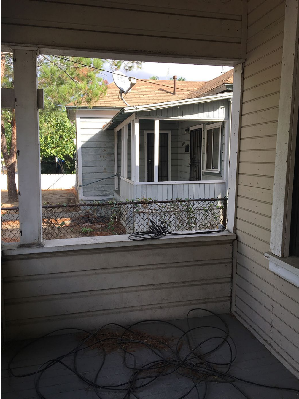
Figure 9 – Porch detail, view looking north
