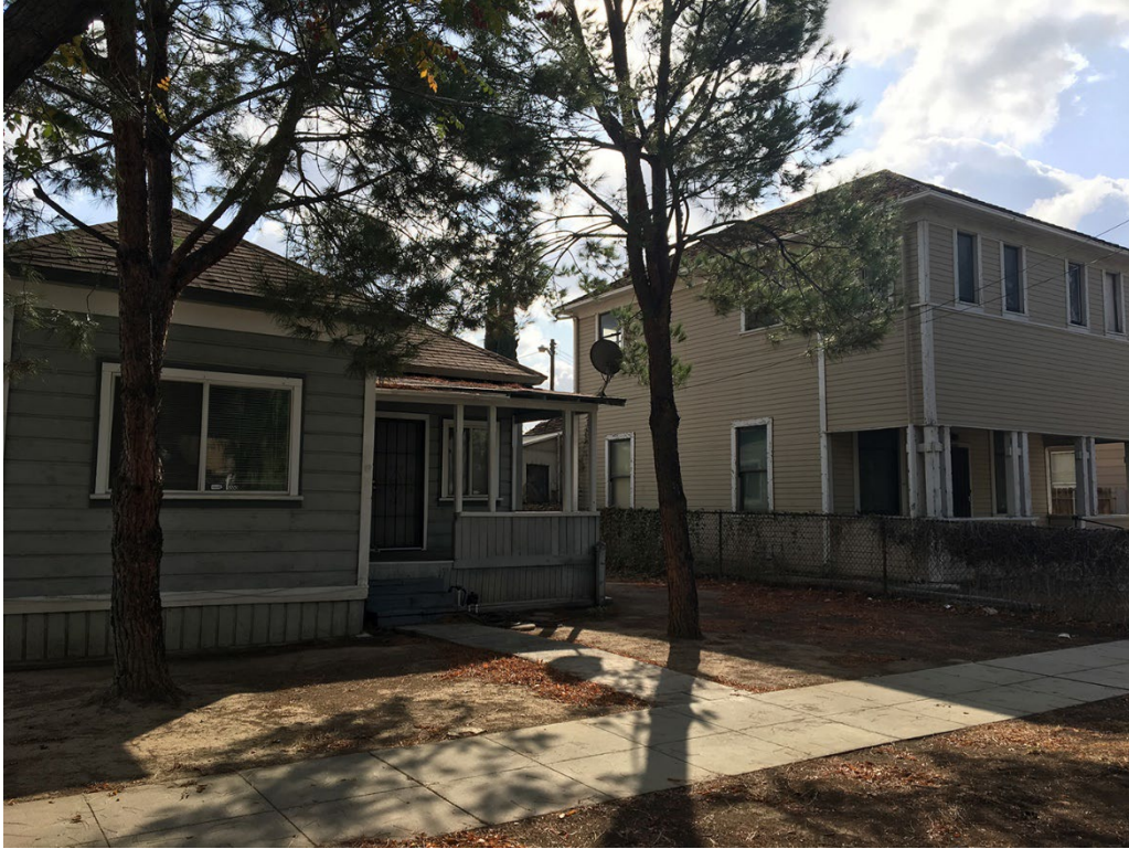
Figure 3 - Harada Hose west and north elevations, view looking southeast
