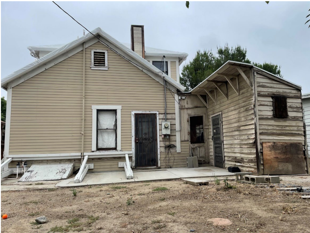
Figure 6 - Harada Hose east (rear) elevation, view looking west
