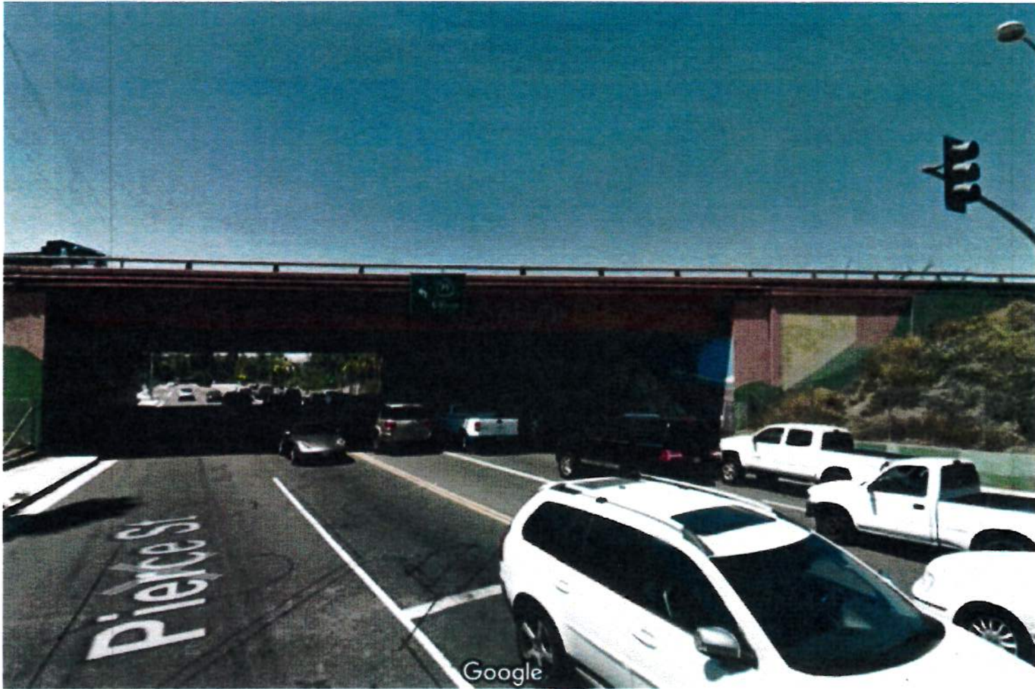
PIERCE STREET UNDERCROSSING
