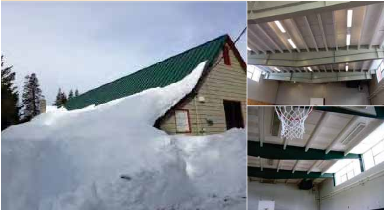
Clockwise from left: Donner Trail Elementary School from the outside; the interior of the roof before it was renovated to meet local building code specifications; the interior of the roof after it was renovated to meet building code requirements.
