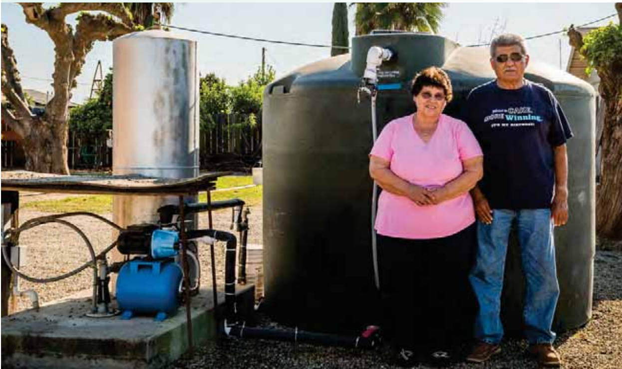
Project in the unincorporated community of Monson
