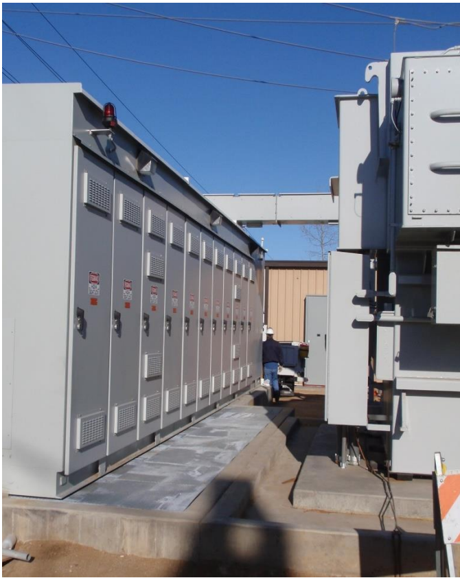
Proposed new transformer and switchgear equipment at La Colina Substation
