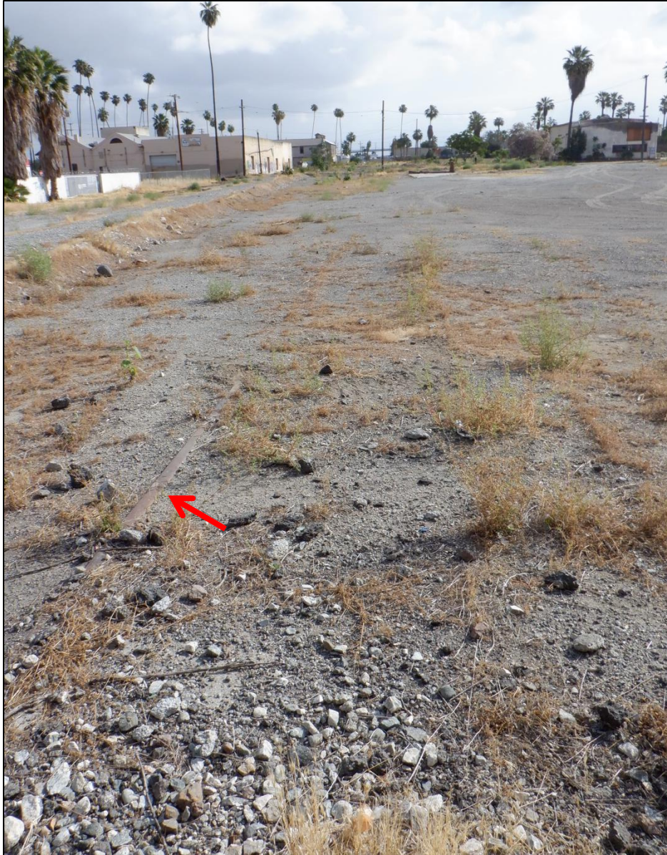
Figure 13. Partially exposed rail southeast of 3093 Mission Inn Avenue, facing south.
