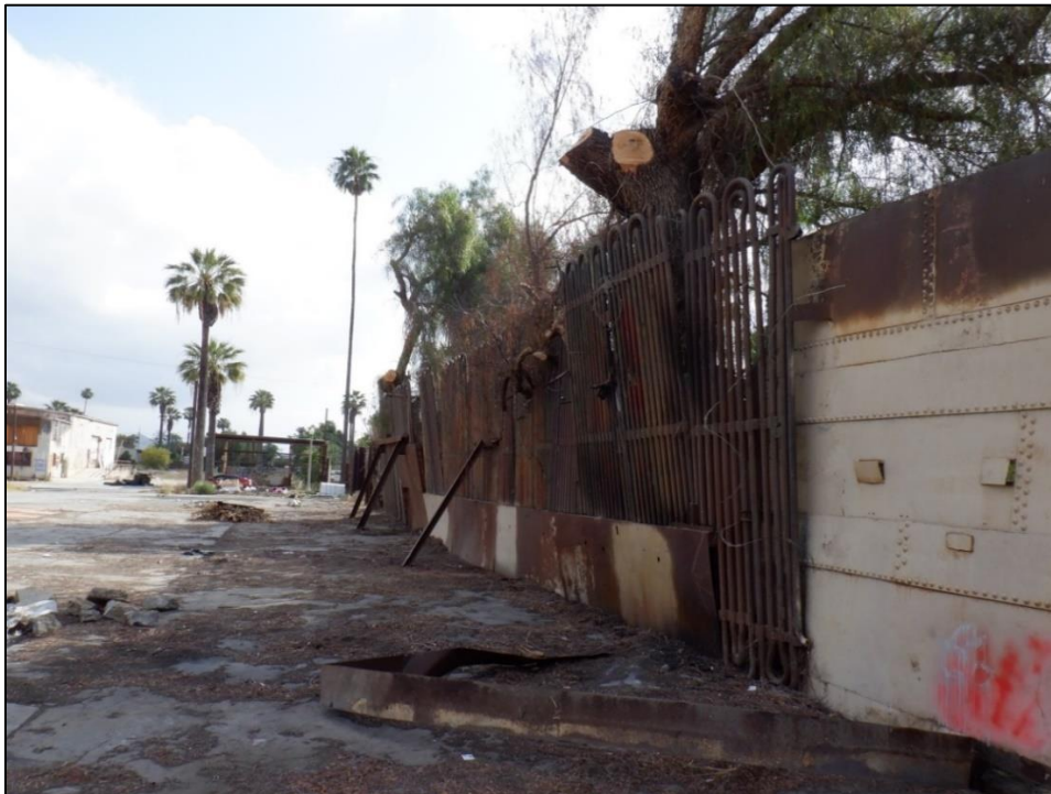
Figure 17. Coils located between Mission Inn Avenue and 6 th Street, facing northeast
