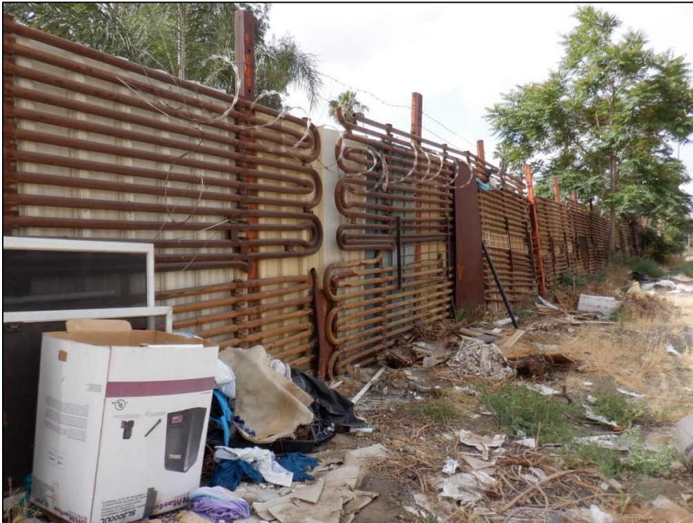
Figure 19. Coils located between 6 th Street and 5 th Street, facing southwest
