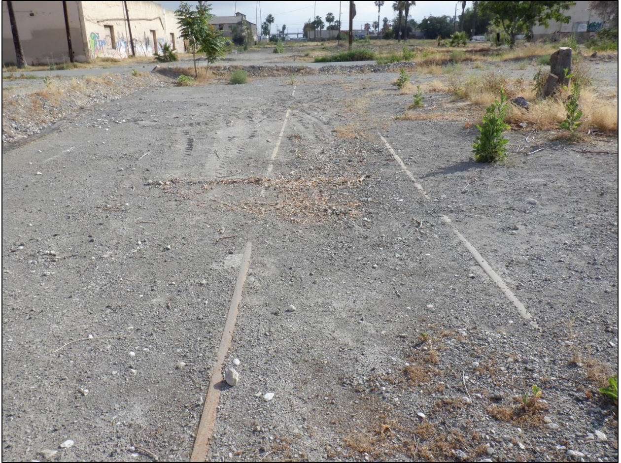
Figure 14. Partially exposed rail southeast of 3093 Mission Inn Avenue, facing south.
