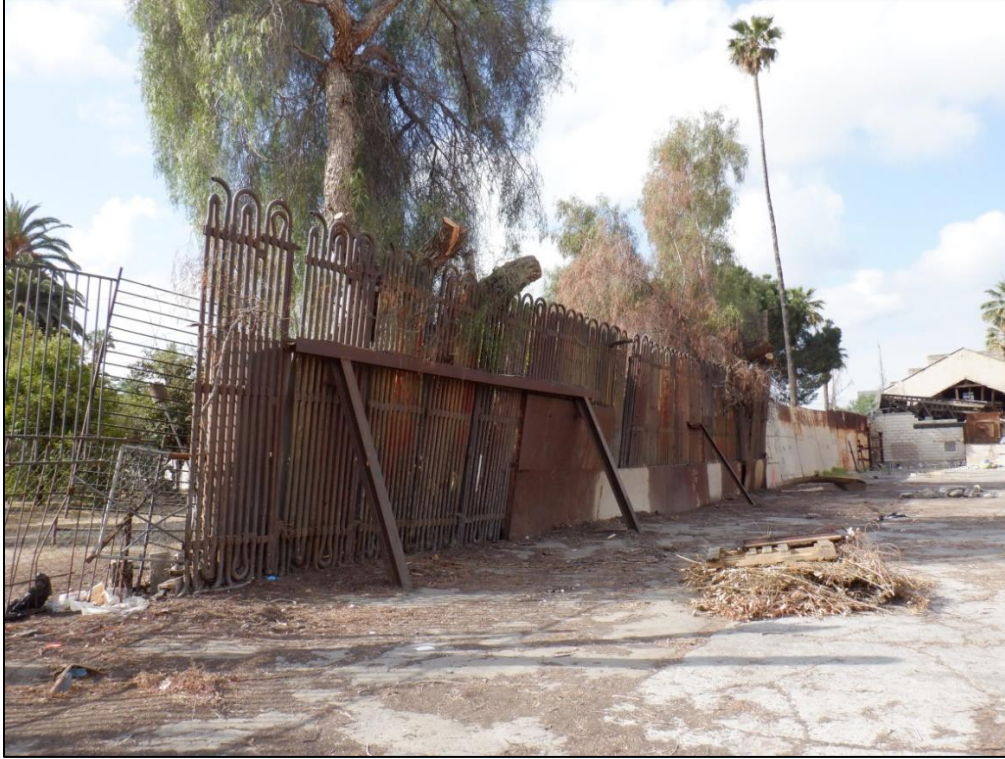
Figure 18. Coils located between Mission Inn Avenue and 6 th Street, facing southwest
