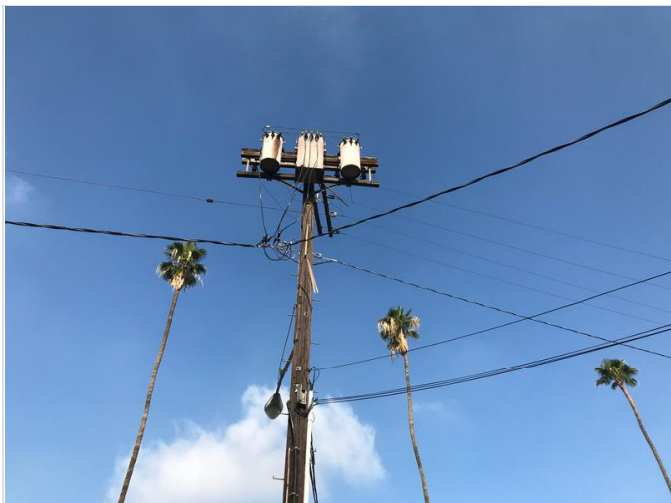
31. Pole-mounted transformers
