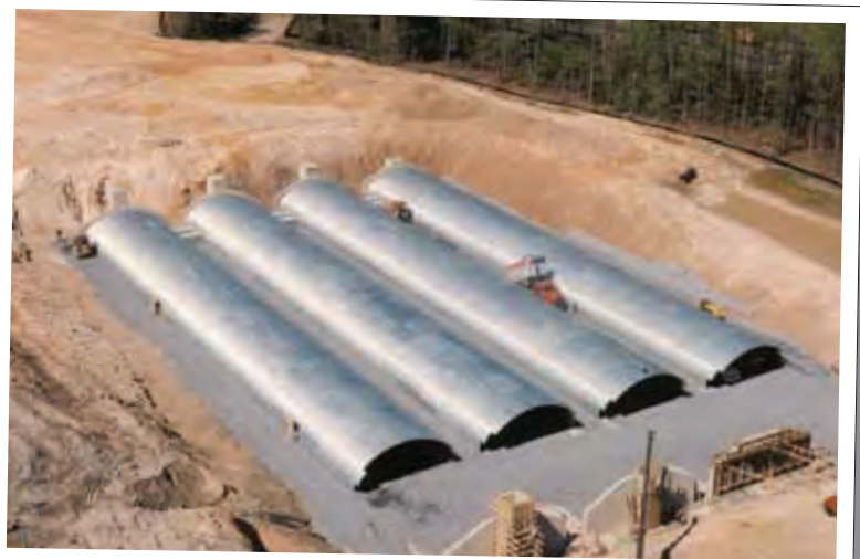
Plate system for high volume storage
