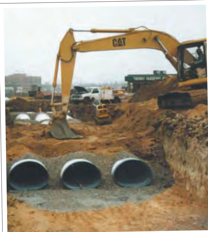
Pipe-arch for low profile application.
