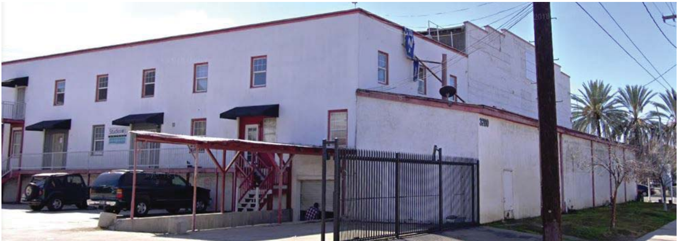
North and west elevations, view looking southeast
