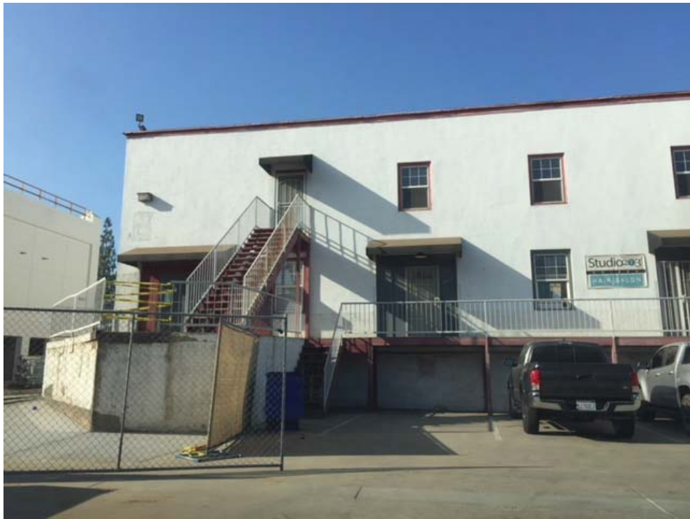
Two-story administration addition, view looking south
