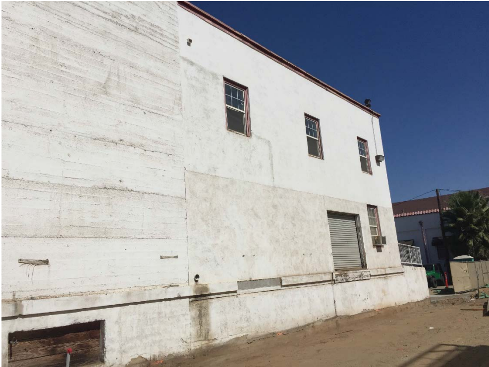
East elevation loading bay, view looking northwest
