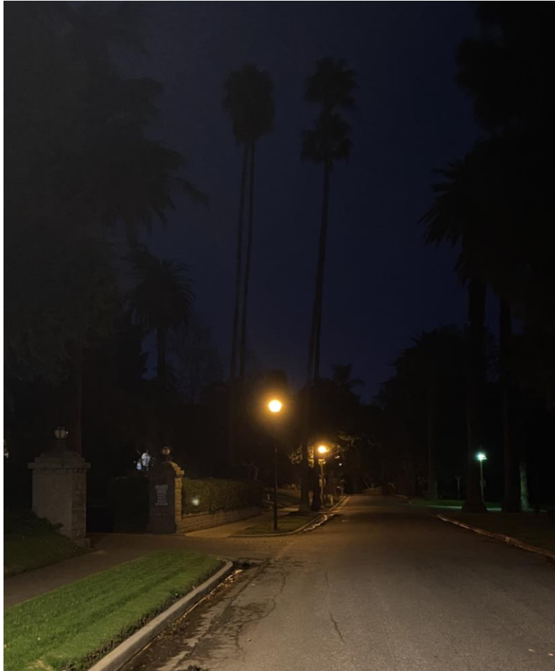
Existing HPS Lamp (1900-2000K) Mt. Rubidoux Drive Ladera Lane - Sixth Street
