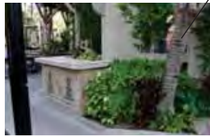
Existing plants to be relocated for new paving and path to wheelchair lift.
