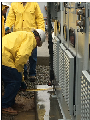
Substation Equipment Upgrades
