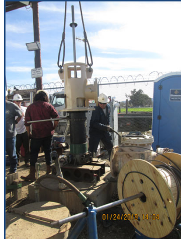
Garner 5 Well – New Column Pipe and Pump
