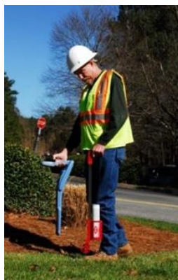
Typical underground facility locating
