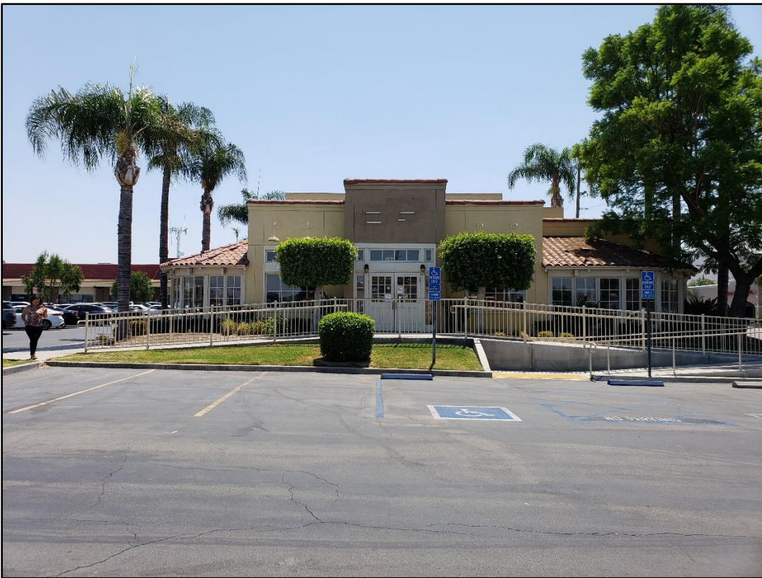
Existing Building to be demolished, looking from within shopping center parking lot PR-2021-001049 (Conditional Use Permit and Design Review) – Exhibit 3 – Existing Site Photos
