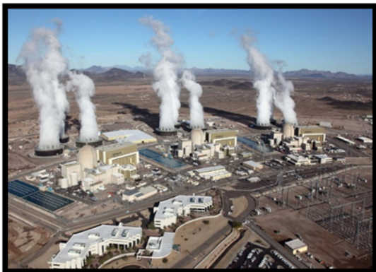
Palo Verde Nuclear Generation Station (1981)
