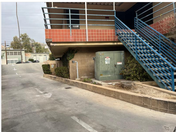
13. Pad-mounted transformer
