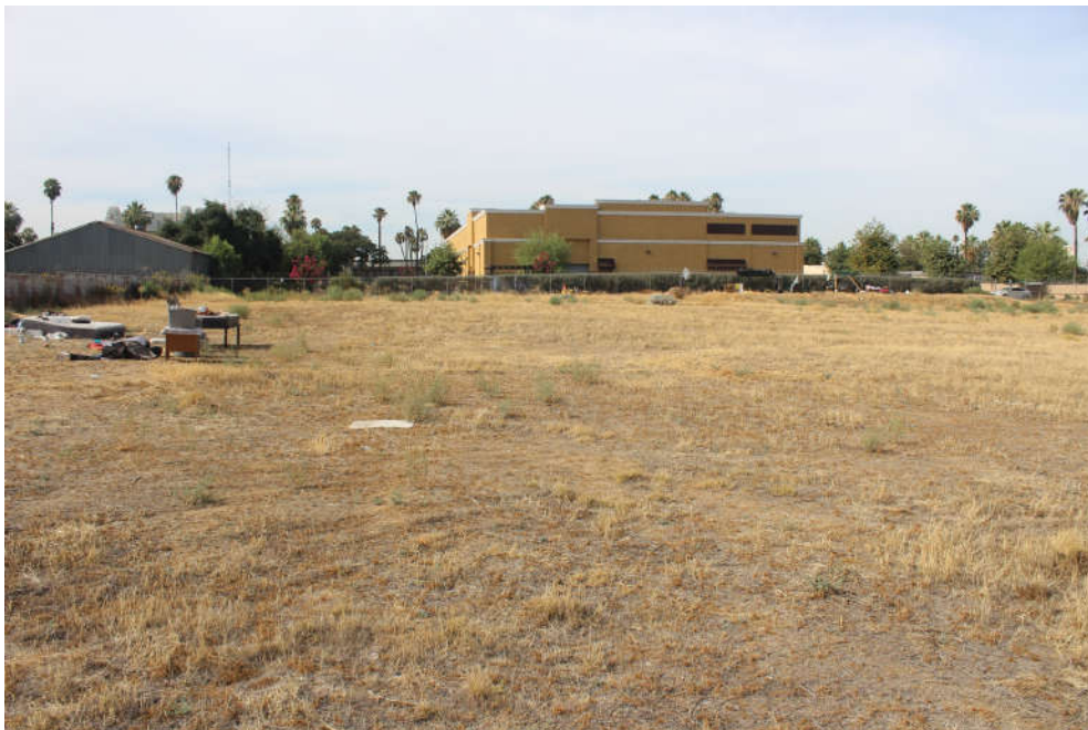
Photograph 2 (S). Photograph depicts the undeveloped portion of the project site with the existing building in the background.
