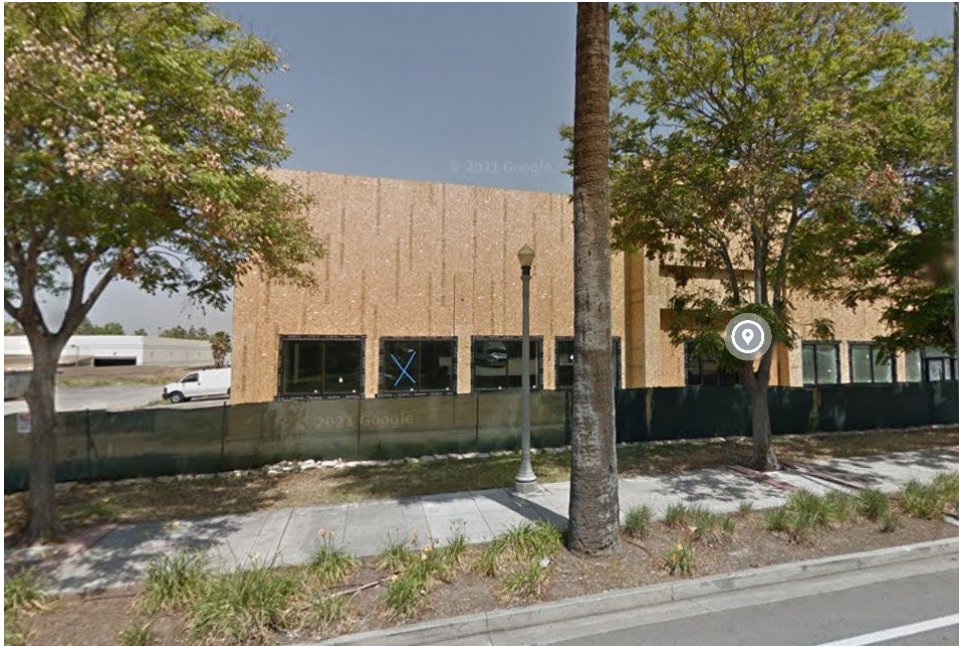
Figure 2: Exterior of Building under Construction in 2015 (Google Maps – Street View)
