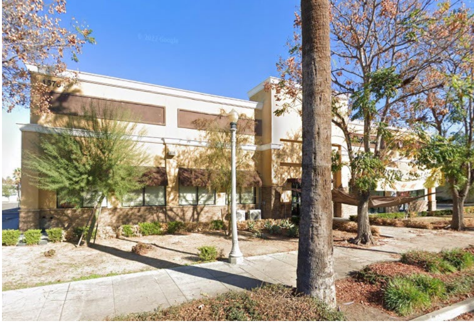
Figure 3: Overview of Modified Exterior in 2022 (Google Maps – Street View)
