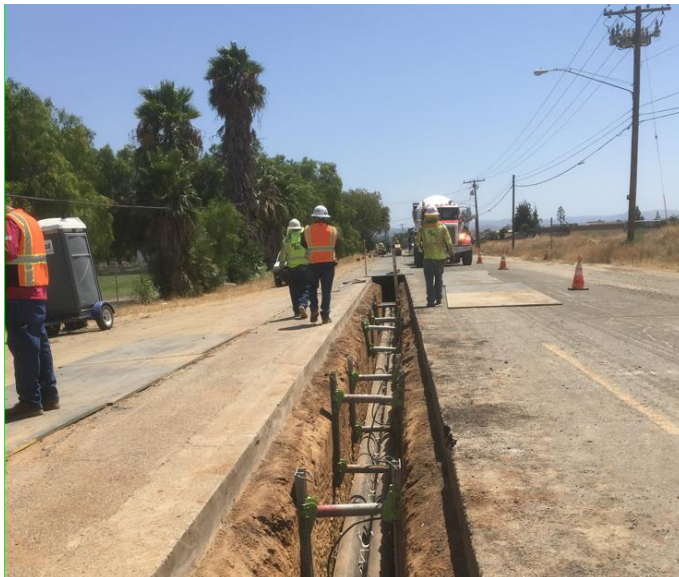
Typical trench/conduit and underground vault installation
