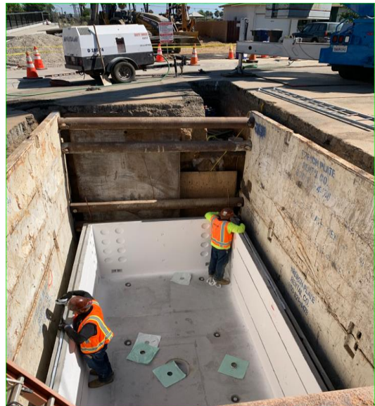
Typical trench/conduit and underground vault installation
