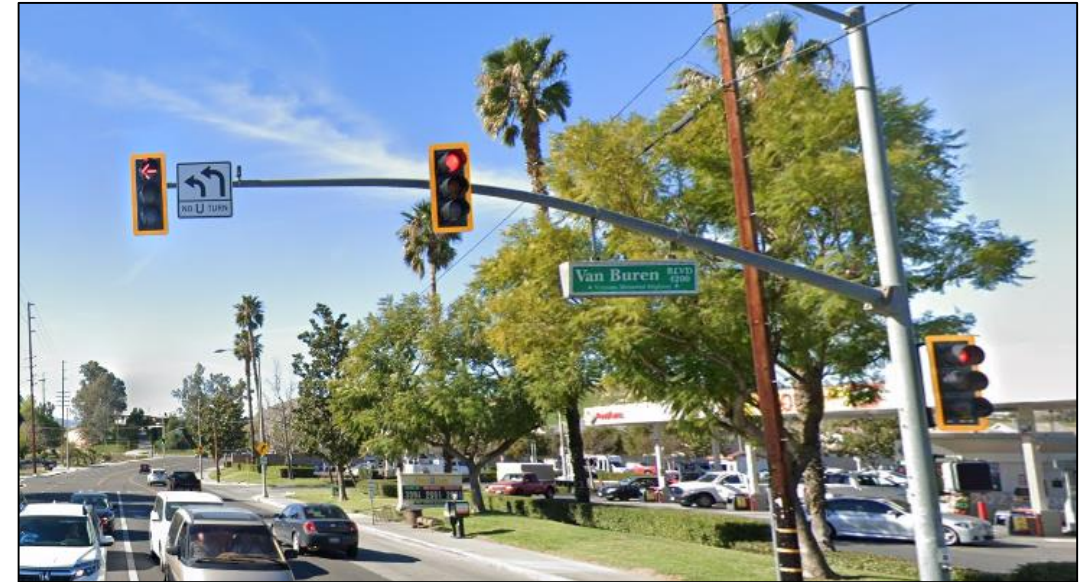
Install retroreflective backplates to increase visibility of signals
