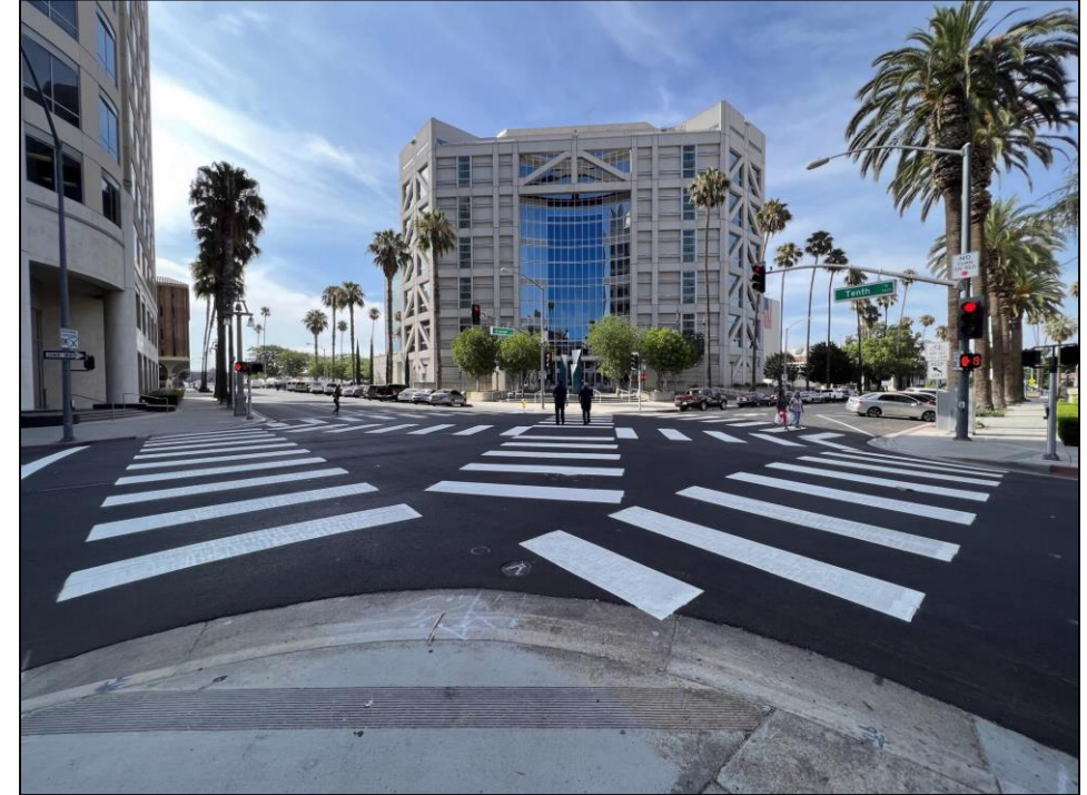
Install continental crosswalks
