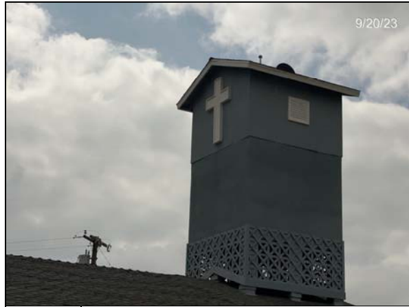
20. North/West Side Steeple
