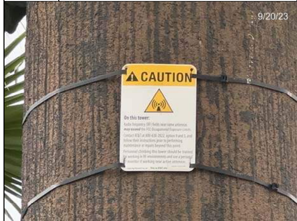
4. AT&T Caution Signage
