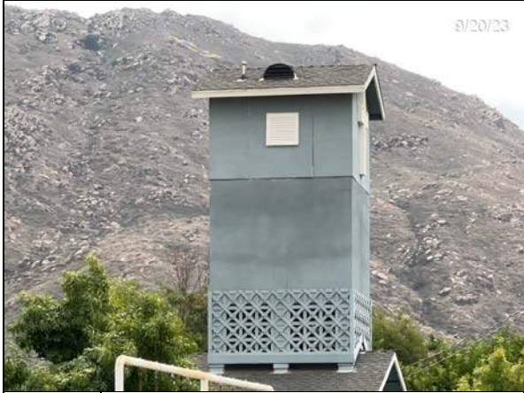
18. View of West Steeple
