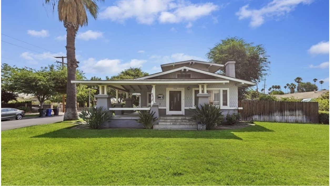
Figure 1 - Front Facade (west elevation), looking east
