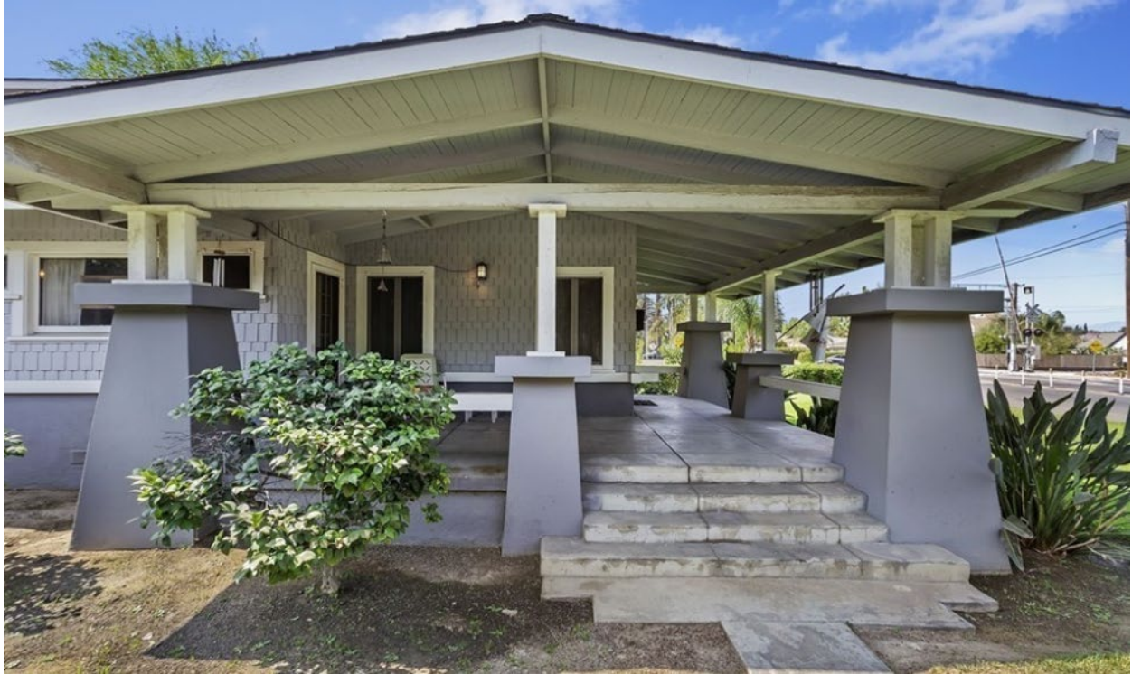
Figure 3- Front Porch, looking south
