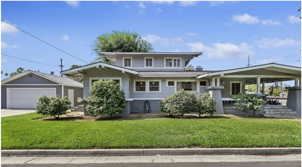
Figure 2 - North Elevation, looking south
