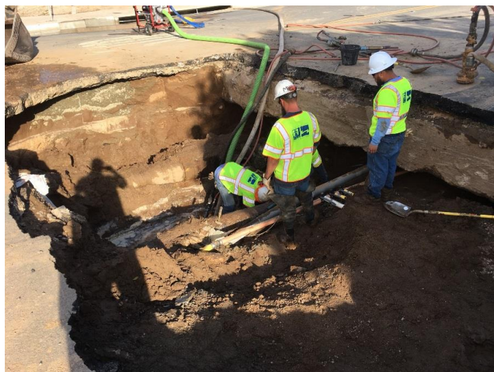
Figure 2 - Repairing the pipe
