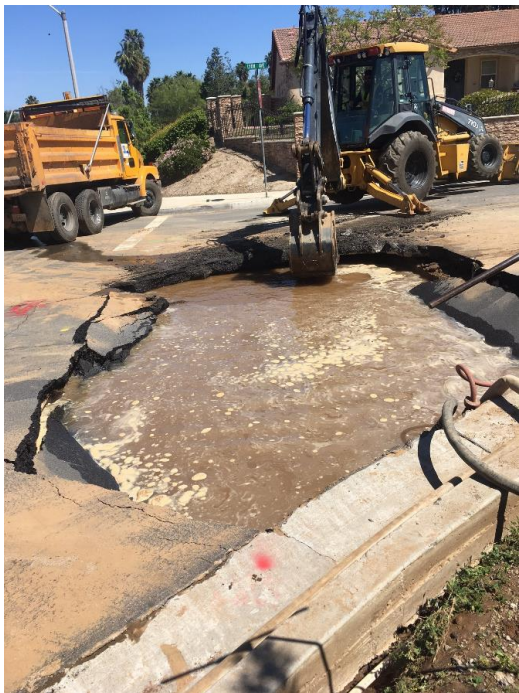
Figure 1 - Excavating the pipe
