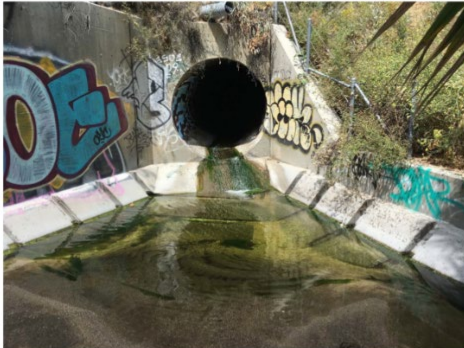
Fig 2: Western entrance to the (approximately) 450-foot-long 5-foot diameter culvert under I215 freeway that is a non-feasible option for creating Constrained Linkage 7. (photo June 2019 LN)
