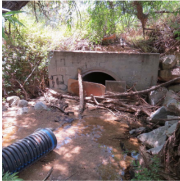
Fig 3: Southern entrance to the (approximately) 250-foot-long 5-foot diameter culvert under Central Ave that is a non-feasible option for creating Constrained Linkage 7.
