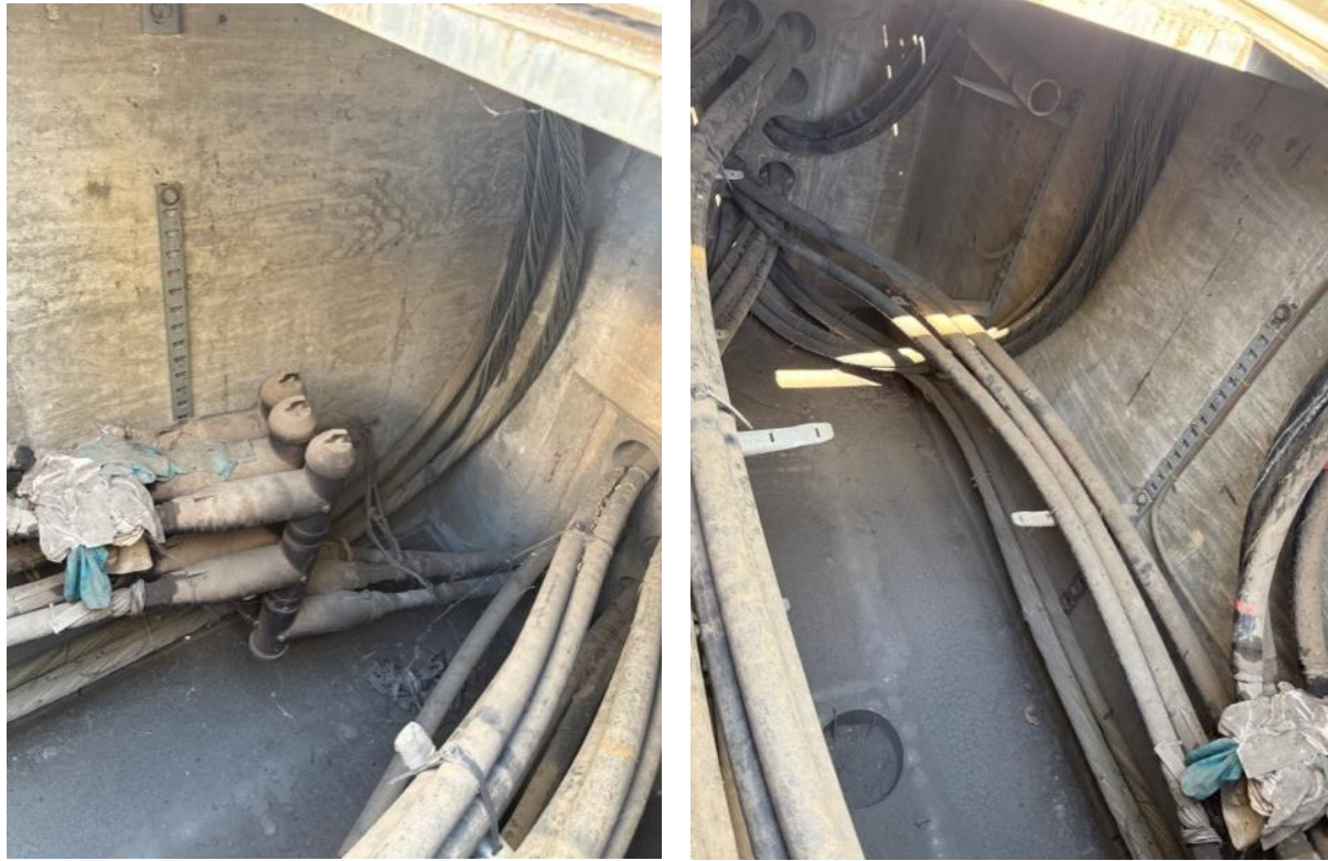
Underground Primary Feeder Cables at the Substation Cable Pit
