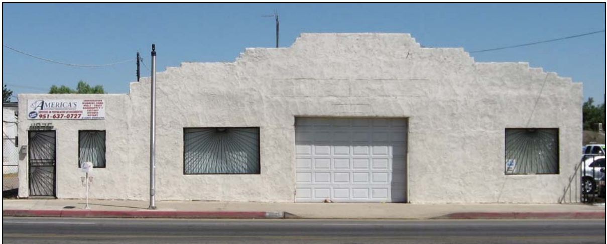
Figure 29. 11075 Hole Avenue, view to the north (2007).
