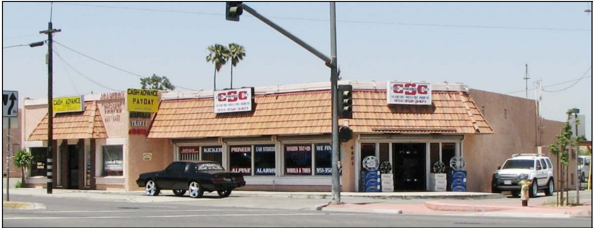
Figure 28. 5901-03 La Sierra Avenue, view to the northeast (2007).
