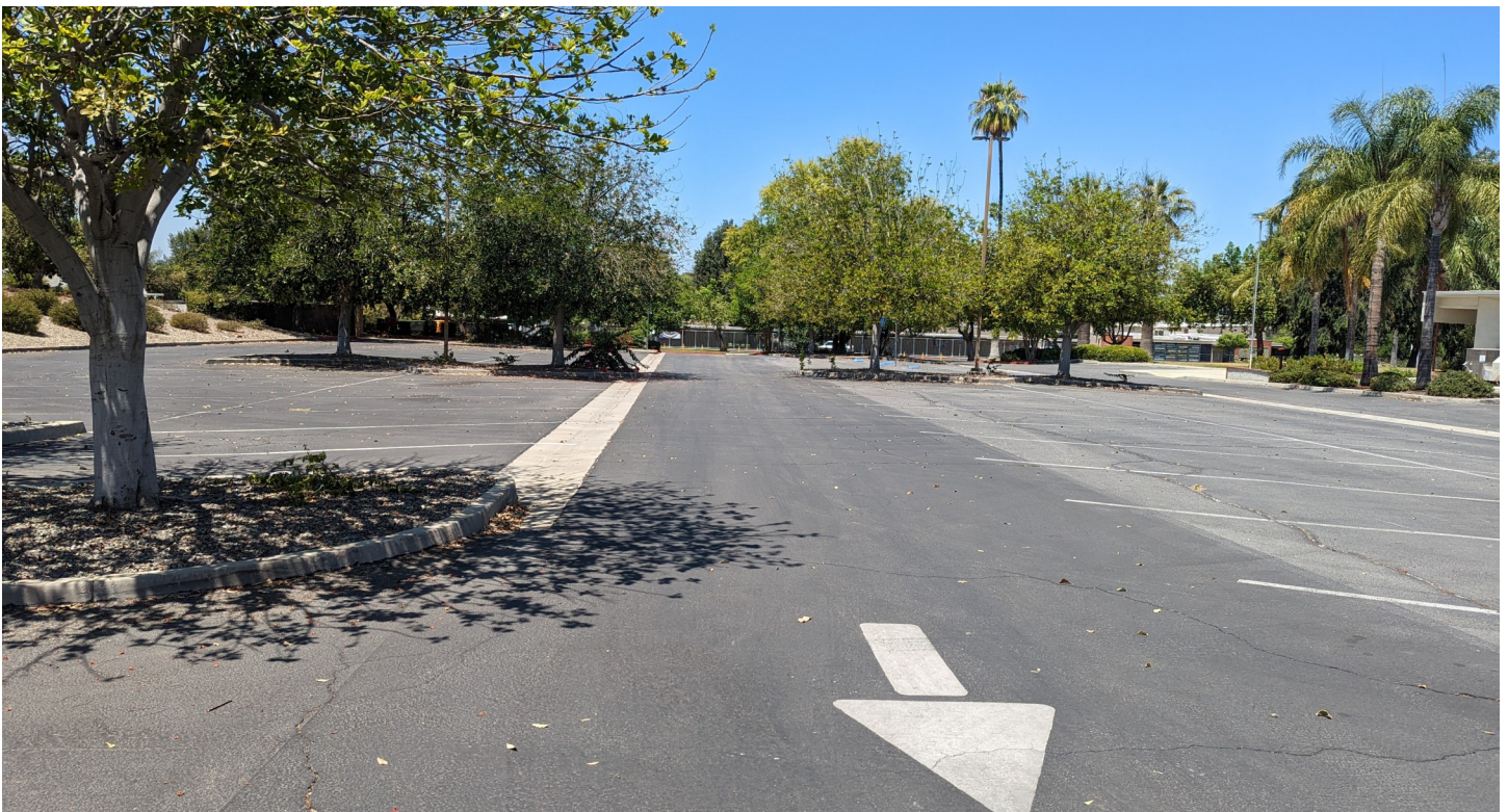
View of the parking lot looking west
