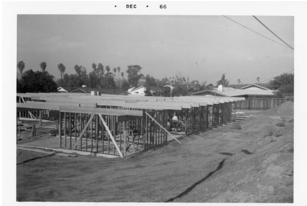
Rear/east side elevations, 1966
