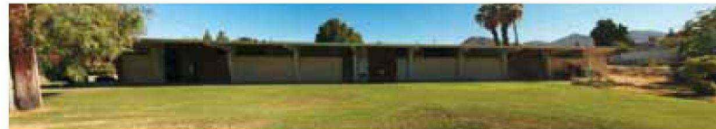
(E) CLASSROOM BUILDING SOUTH FACE
