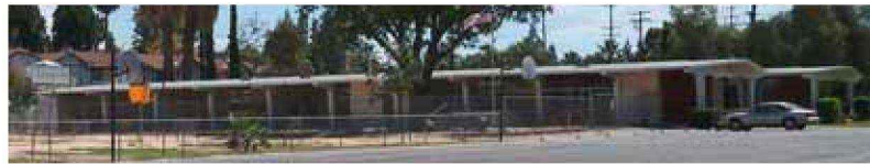
(E) CLASSROOM BUILDING NORTH FACE
