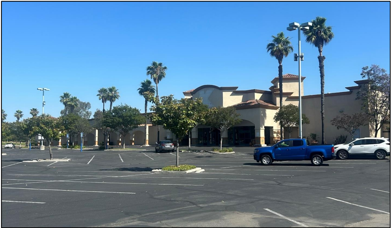
View of the existing site looking south from the parking lot.
