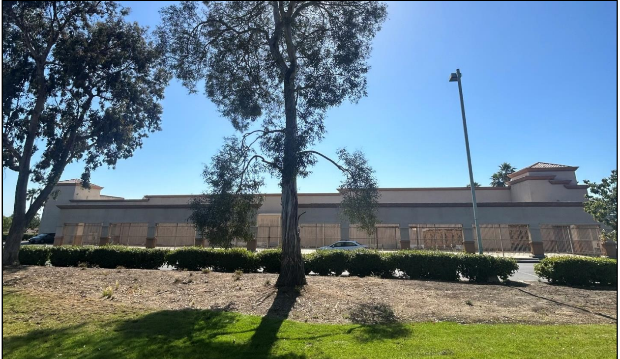
View of the existing site looking north from Mission Village Drive.
