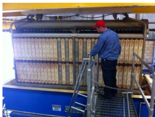
Ultrafiltration Basin (Train No.5) Cassette removal for inspection
