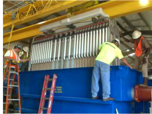
Cassette removal for inspection
