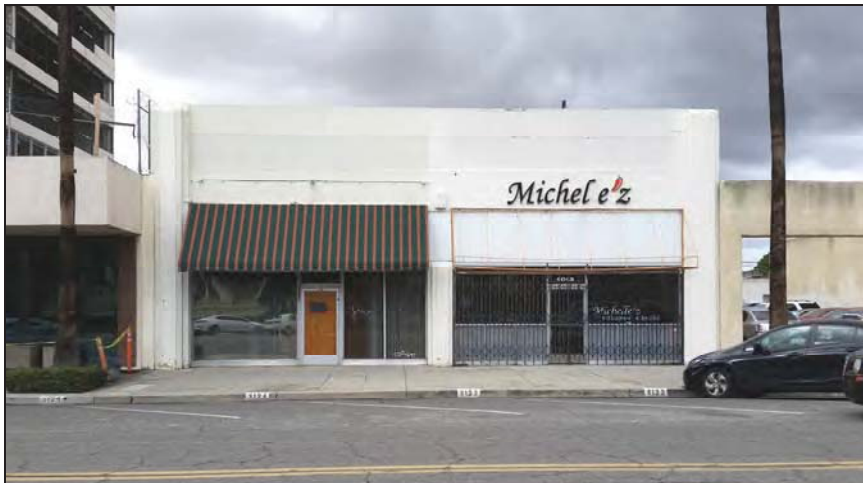
4049-4053 Main Street. View to the northwest (January 7, 2016)
