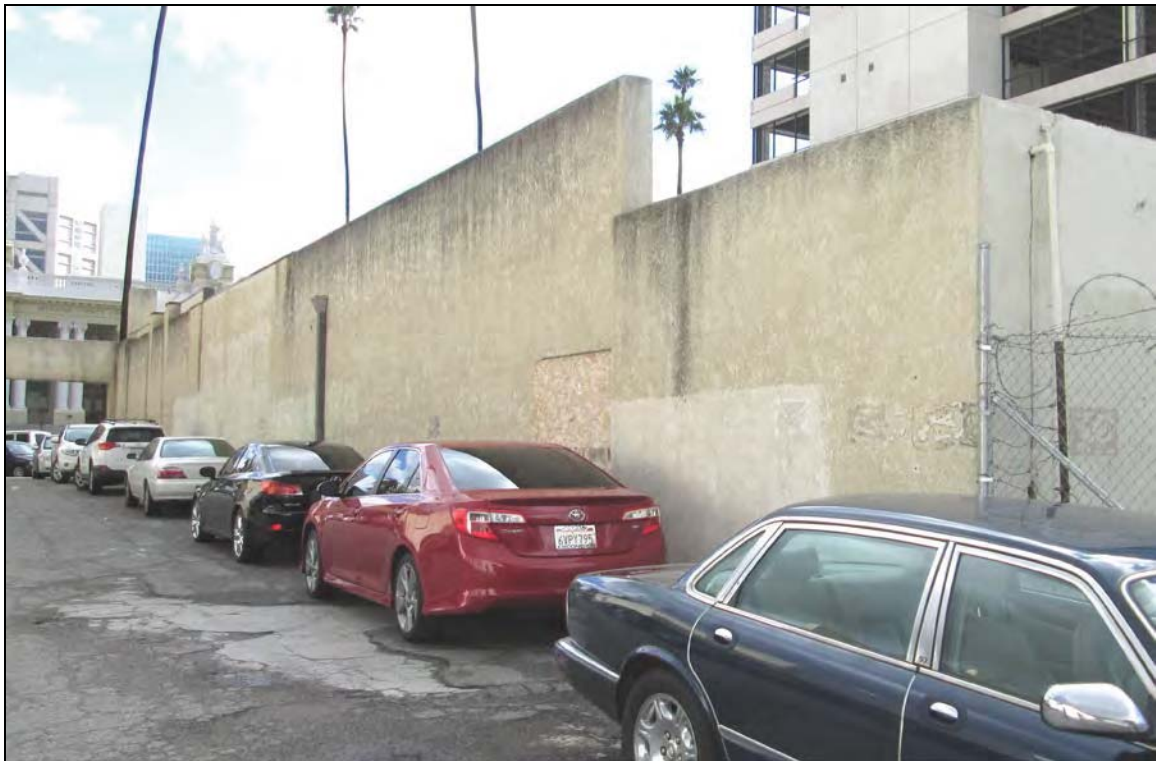
Figure 5 – North elevation, view to the southeast (1/7/2016)
