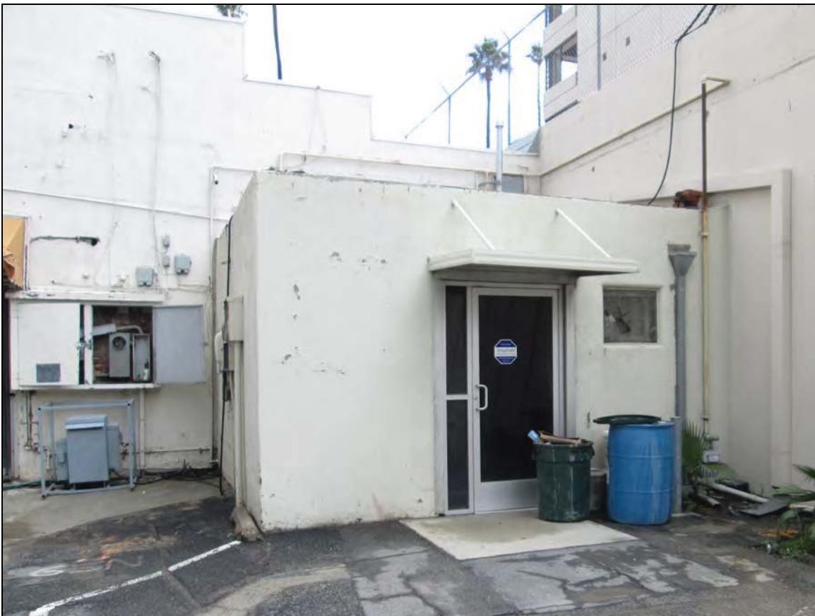
Figure 7 – Smaller rear addition, view to the southeast (1/7/2016).
