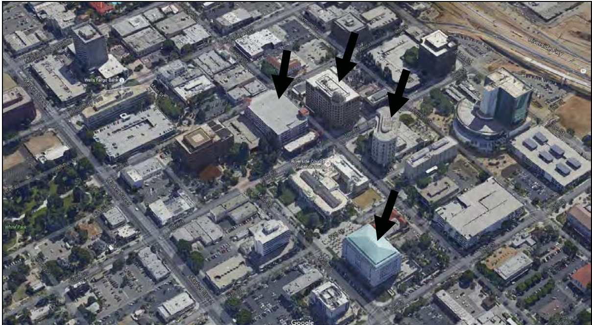
Figure 11 – Aerial image showing the project vicinity and the four multi-story buildings near the Courthouse. (Source: Google 2016)
