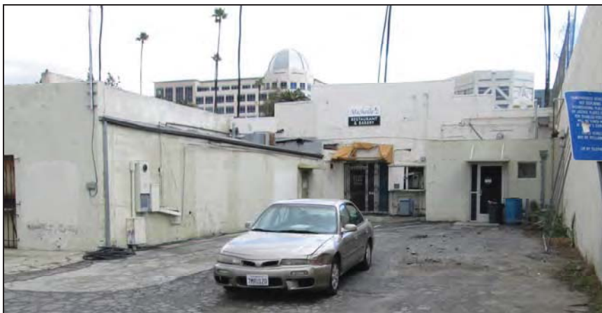
4049-4053 Main Street. Rear of the building (January 7, 2016)
