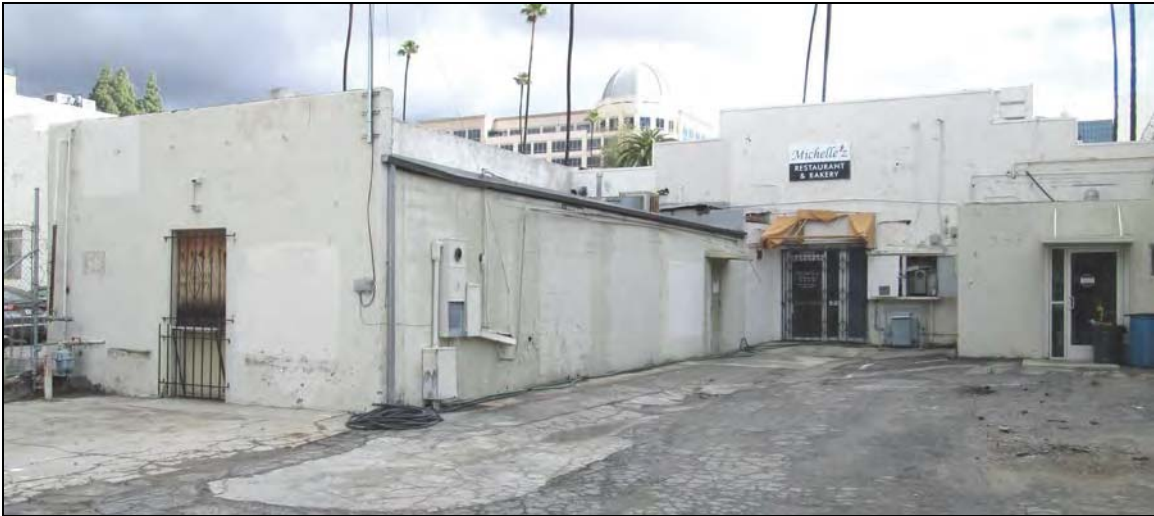
Figure 6 – West (rear) elevation, view to the east (1/7/2016).
