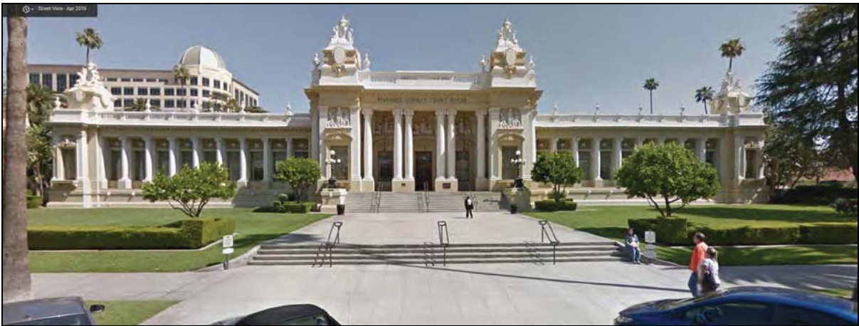
Figure 15 – County Courthouse, 4050 Main Street. View to the southeast. (Source: Google April 2015).
