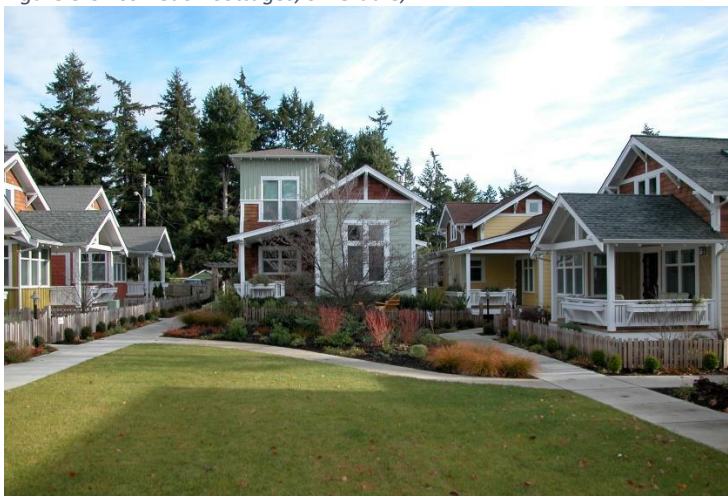
Figure 9 Ericksen Cottages, Bainbridge Island, WA
