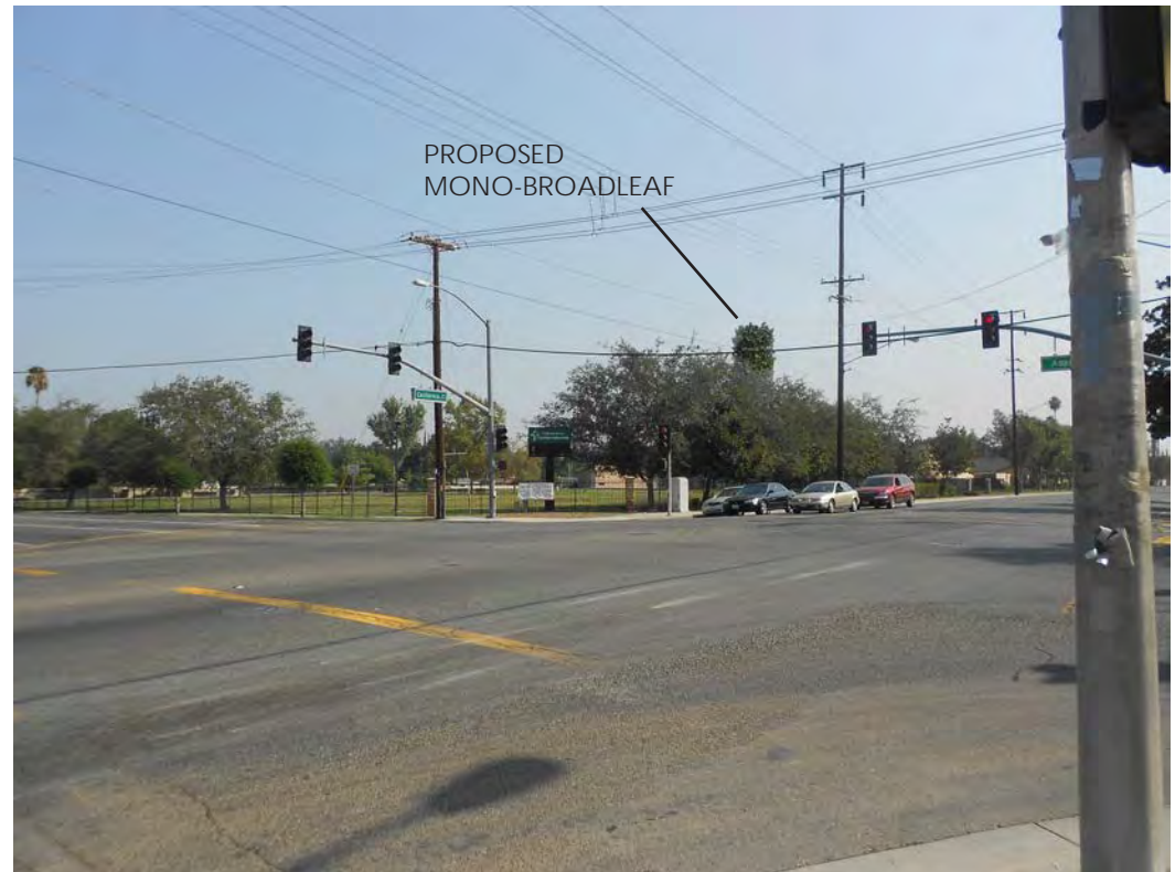
PROPOSED INSTALLATION OF 60' MONO-BROADLEAF WITH VERIZON ANTENNA ARRAY AND TWO (2) PARABOLIC ANTENNAS. INSTALLATION OF EQUIPMENT COMPOUND/TRASH ENCLOSURE SCREENED BY A 8' CMU WALL (COMPOUND NOT VISIBLE FROM THIS VIEW).
