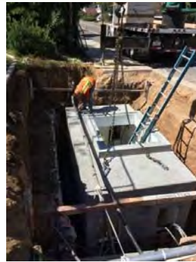
Repair or Replacement of 5 Underground Vaults
