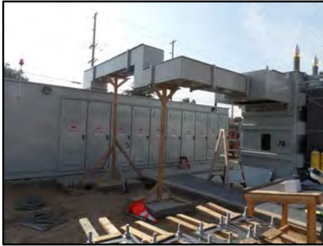
Substation Switchgear Upgrades
