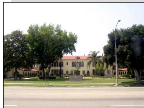
The Palm Elementary School building, which currently houses the Riverside Unified School District's Community Education program, is a designated historic landmark in the Magnolia Center District.
