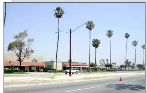
Sporadic parkway landscaping and no median landscaping occur along portions of Magnolia Avenue.
