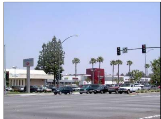
The intersection at Magnolia Avenue and Tyler Street could be improved for both pedestrians and drivers with improved signage, parkway landscaping, and enhanced crosswalk and intersection paving.
