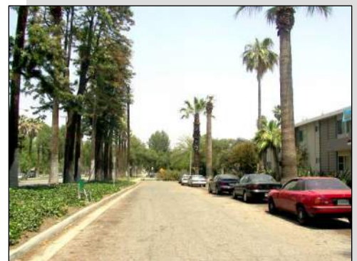
Frontage roads adjacent to Magnolia Avenue have disrupted the historic parkway landscaping in parts of the District.
